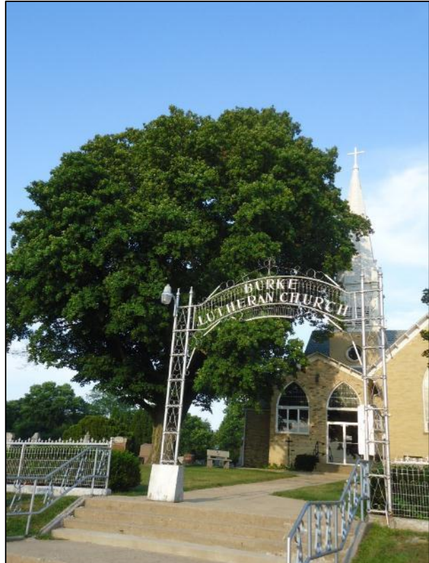
Burke Lutheran Church is and will continue to be a recognizable place within the community, photo courtesy Mead & Hunt, Inc. 2013
