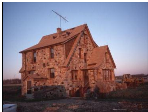
The Lucinda and Samuel Messerschmidt House, built in 1930 is a Tudor Revival style and has been determined eligible for the National Register of Historic Places. Source: Wisconsin Architecture and History Inventory
