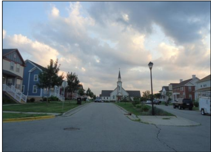
Institutional land uses, like the church shown above in the City of Sun Prairie "Providence" planned neighborhood, provide key focal points within traditional neighborhood developments. Photo courtesy Mead & Hunt, Inc., 2013
